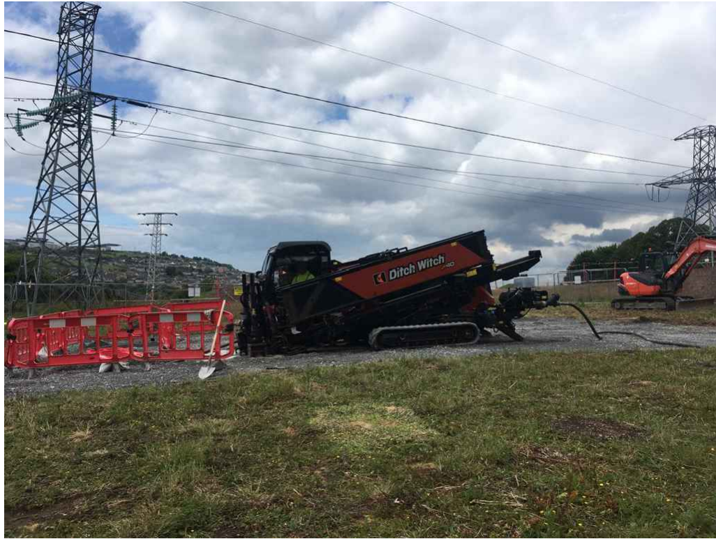
Image 1 : Directional Drilling Rig
